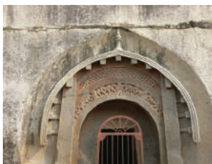
Mauryan Structure at Barabar Caves
