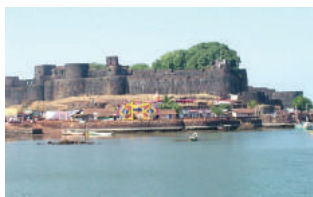
Vijaydurga Fort, Sindhudurg
